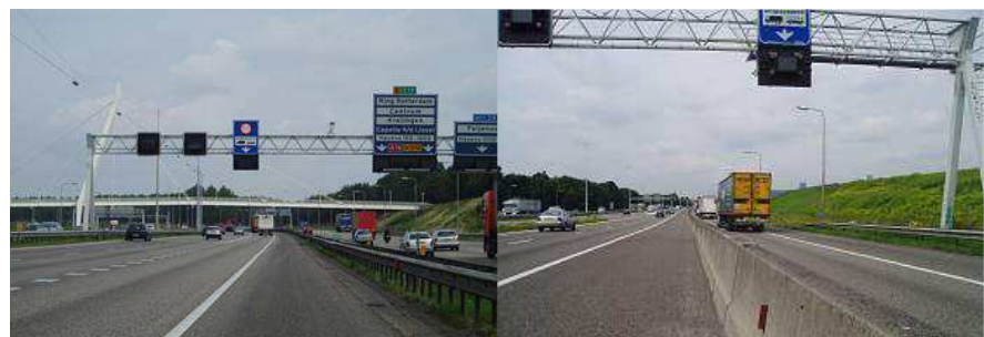
(a) Non-physically separated truck lane on the A16 (b) Physically separated truck lane further downstream on the A20
