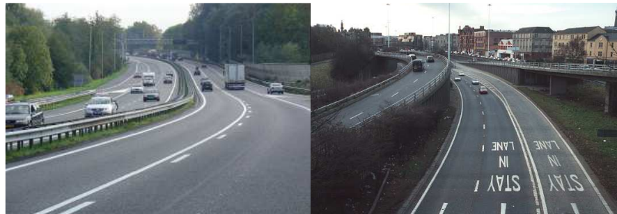
(a) Solid marking along an on-ramp in the Netherlands (From: Eindboek FileProof)
