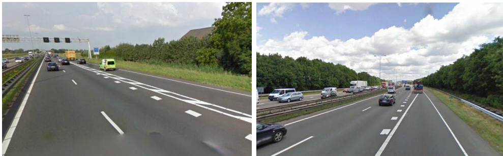
Figure 7.13: Layouts of the A50 section. On the left the start of the section, on the right the end of the section
