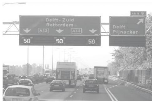
..... Figure B.7: Illustration of Dynamic Speed Harmonization
